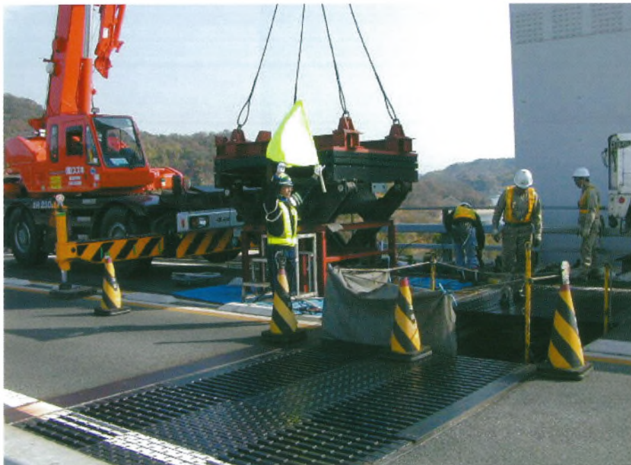
伸縮装置設置状況 Installation of expansion joint
