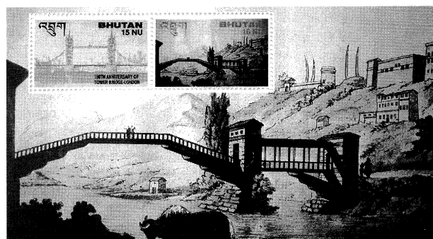
Wangdue Zam (bridge) span of 180 ft. long, constructed with timber without using single piece of iron, built in mid eighteenth century, was maintained for public use till damaged by flood in 1968.
