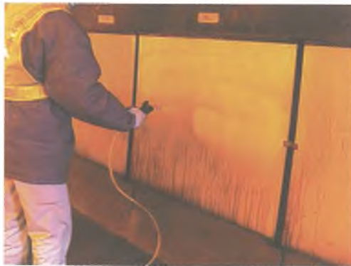
写真-6 内装板の洗浄実験 Photo.6 Cleaning test on side panel
