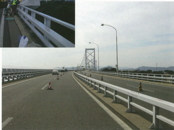
写真一4 撤去完了 Photo.4 After removal
