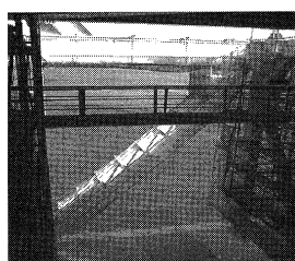
写真-8 主横改良足場 Photo.8 Improved scaffolding for main girders
