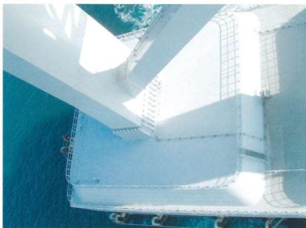
写真-1 頂版部一部ライニング完了 Photo 1 Finished part of resin-paint coating
