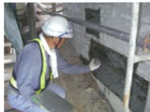
写真-6 断面修復状況 Photo.6 State of Section Remedy
