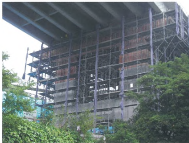
写真-8 3P 施工状況 Photo.8 Working Situation (3 P)
