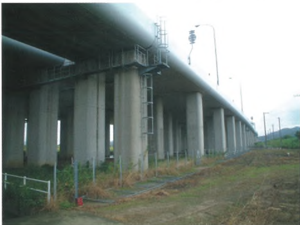
写真-3 4P付近施工前 Photo.3 Before Retrofitting (4 P)
