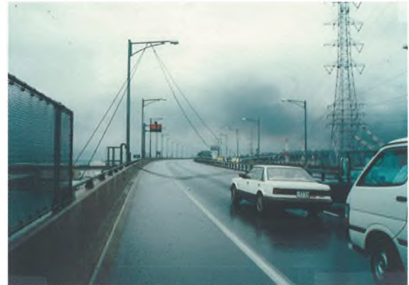
巻頭写真-14 坂出北 IC 付近四国電力送電鉄塔倒壊による交通阻害 (1998) Opening photo.14 Shutting down by the collapse of power transmission tower around Sakaide-Kita Interchange ※ P 9 参照 (See page 9.)
