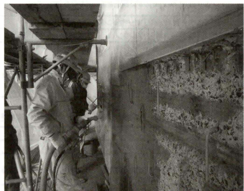
写真-6 断面修復工の施工状況 Photo 6 Patch repair work
