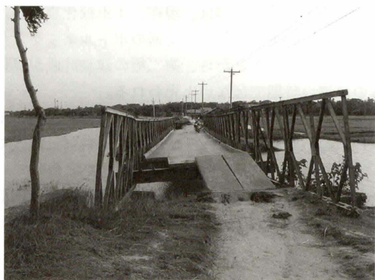
写真-3 洗掘により崩壊寸前のRC橋（仮設のベイリー橋） Photo 3 A RC bridge about to collapse (A temporary Bailey bridge was constructed over it)
