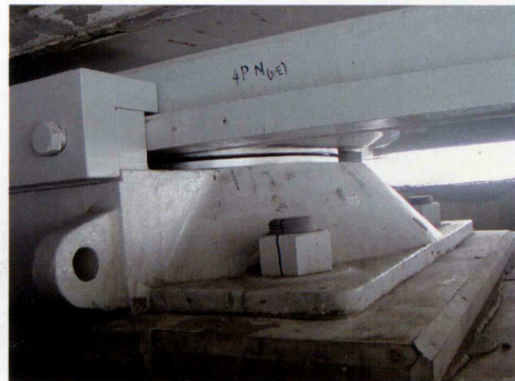
巻頭写真-3 改良すべり板 交換 Opening Photo 3 Replacement of improved slide plate
