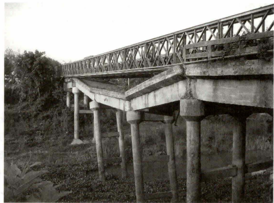
写真-3 洗掘により崩壊寸前のRC橋（仮設のベイリー橋） Photo 3 A RC bridge about to collapse (A temporary Bailey bridge was constructed over it)
