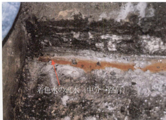
写真-11 目地部 Photo 11 Joint part
