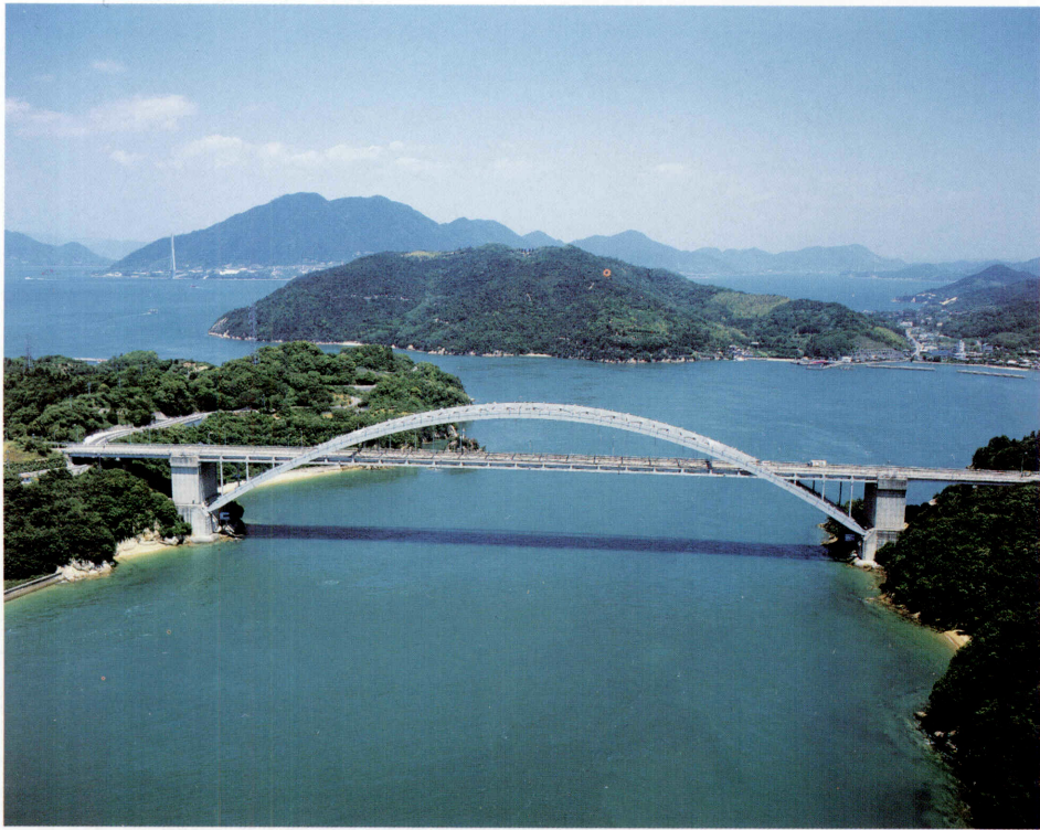
巻頭写真-5 大三島橋 Opening Photo 5 Ohmishima Bridge
