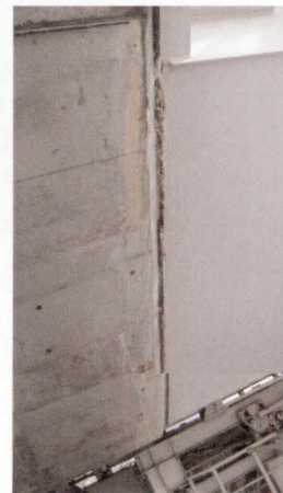
写真-13 接合部桁下状況 Photo 13 Lower part of girder at connections
