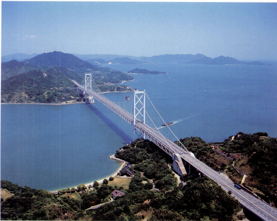
巻頭写真-2 因島大橋 Opening Photo 2 Innoshima Bridge
