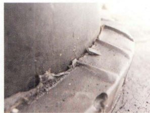
写真-7 隙間1~2mm Photo 7 Gap (1 to 2 mm)
