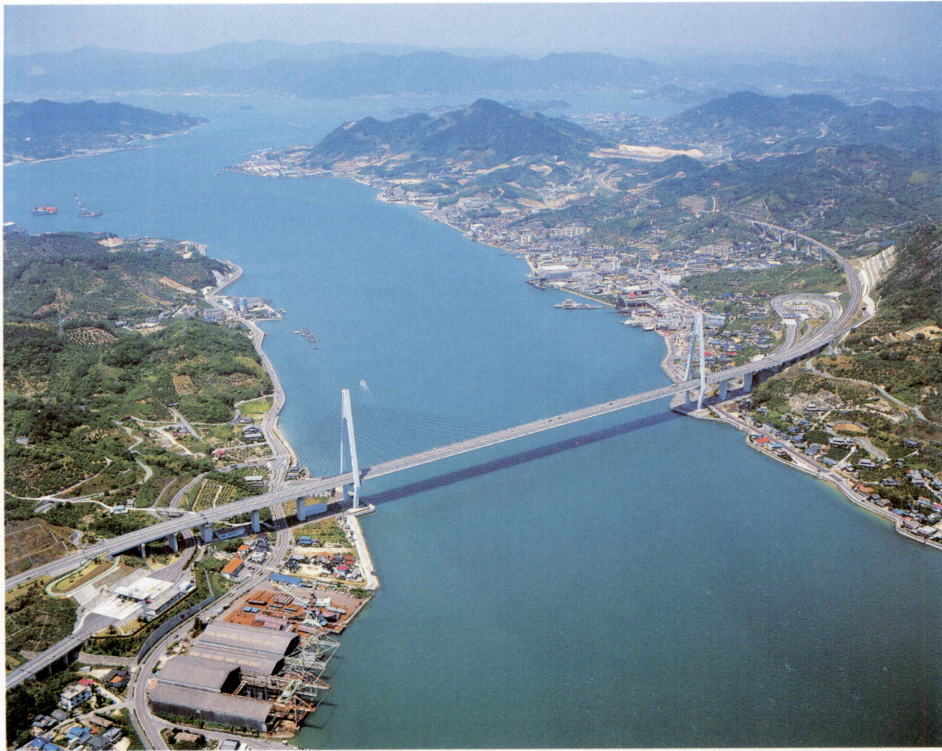
巻頭写真-3 生口橋 Opening Photo 3 Ikuchi Bridge
