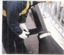
写真-5 雨水対策状況 Photo 5 Countermeasure for rainwater
