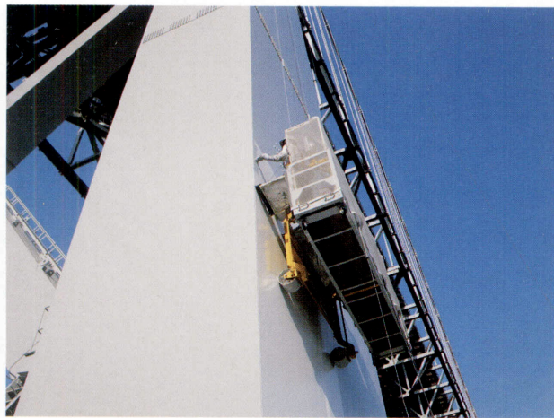
巻頭写真-10 因島大橋3P 東塗装 (上塗り) Opening Photo 10 Recoating on the eastern shaft of Innoshima Bridge 3P
