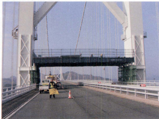
写真-5 路面防護工 Photo 5 Protection work for vehicles
