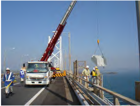
写真-7 架設作業① Photo.7 Setting work
