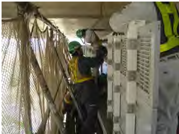
写真-2 施工状況 Photo 2 Construction situation
