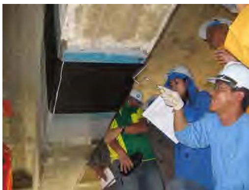
写真-8 炭素繊維補修工事訓練 Photo 8 Field Training of Bridge Repair of Application of Carbon Fiber Sheet
