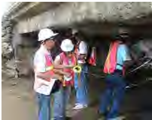
写真-7 橋梁点検訓練 Photo 7 Field Training of Bridge Inspection
