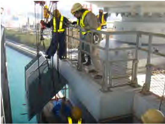
写真-8 架設作業② Photo.8 Setting work
