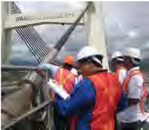
写真-3 点検訓練 Photo 3 Field Training of Bridge Inspection
