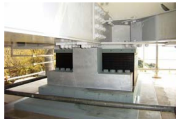
写真-9 支承取替 Replacement of the bearings (2P)
