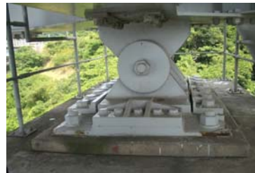
取り替え前 Before replacement
