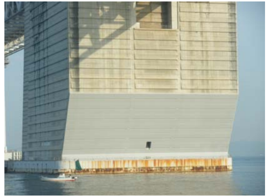
写真-7 南備讃瀬戸大橋7A南面完成 Completion of painting at 7A anchorage
