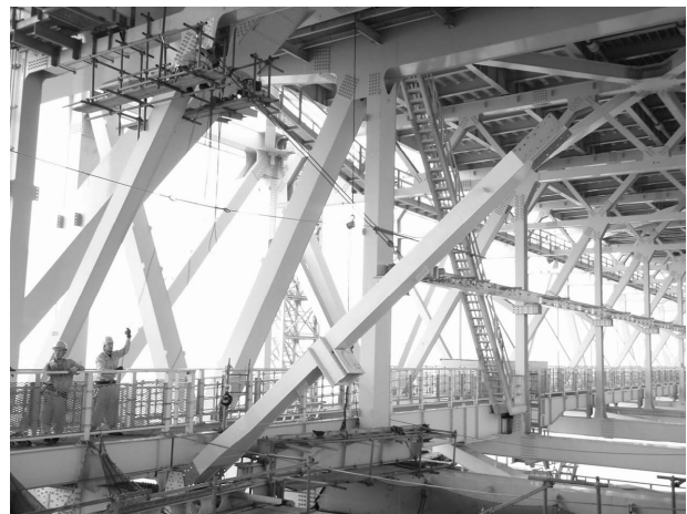
写真-6 垂直材設置状況 Photo 6 The installation of the vertical beam
