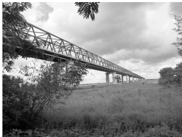
写真-7 Bomyatun 橋 Photo 7 Bomyatun Bridge
