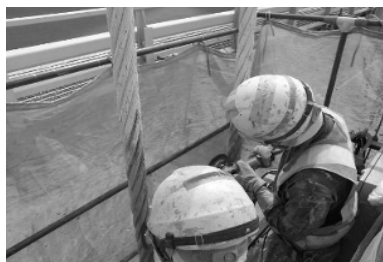
写真-2 飛散防止対策 Photo 2 Countermeasure against dust scattering
