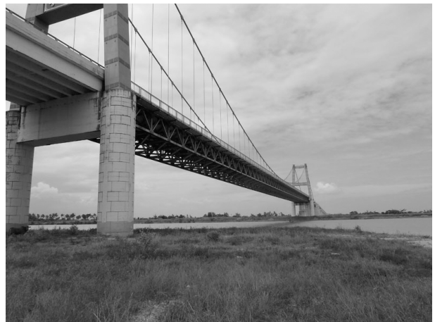
写真-4 Twantay 橋 Photo 4 Twantay Bridge
