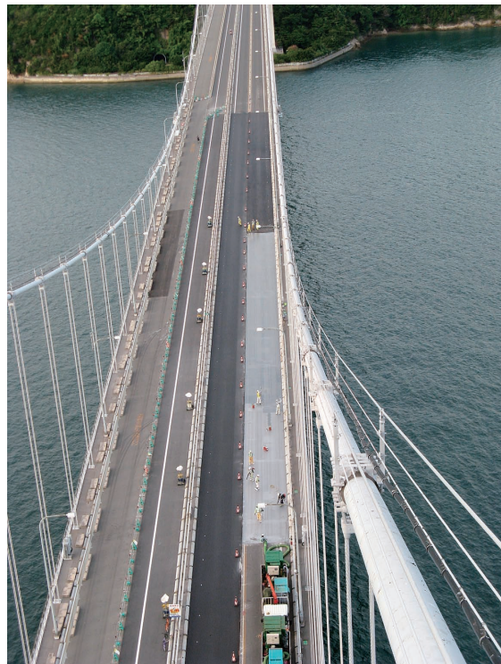
写真-8 橋面舗装打換え状況(接着層工) Pavement replacing work
