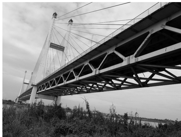
写真-12 Alngzaya 橋 Photo 12 Alngzaya Bridge
