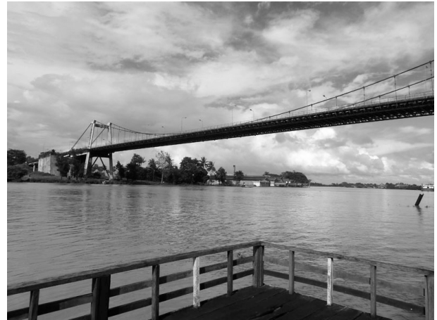
写真-2 Myaungmya 橋 Photo 2 Myaungmya Bridge
