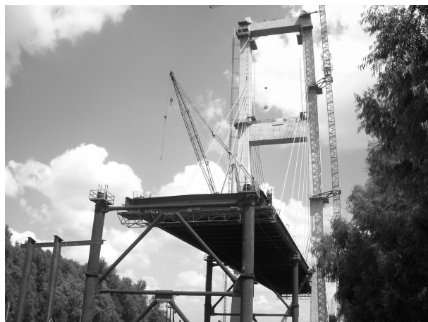
写真-2 John James Audubon Bridge
