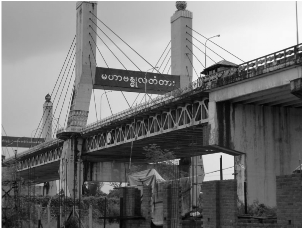
写真-14 Mahar Bandoola 橋 Photo 14 Mahar Bandoola Bridge
