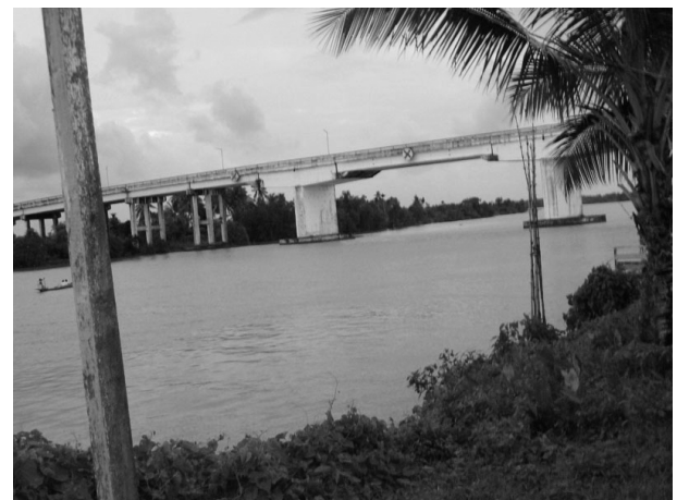
写真-17 Gongyintan 橋 Photo 17 Gongyintan Bridge
