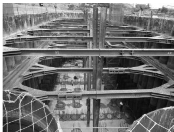
写真-9 底版工完了 (P16) Photo 9 Completion of Bottom Slab (P16)
