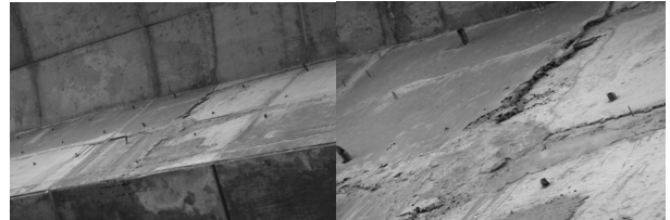
写真-9 取付高架橋の主桁 Photo 9 Main Girder of Approach Bridge
