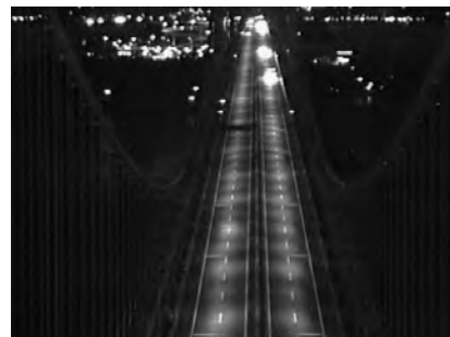
写真-6 BB6Pより北向き映像(夜間映像・既設カメラ) Photo 6 North view from BB6P (Night View・Existing Camera)
