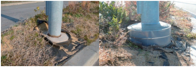
写真-3 コンクリート巻き補修（施工前・施工後） Photo.3 Repair of the Pole Covered by Concrete around the Base
