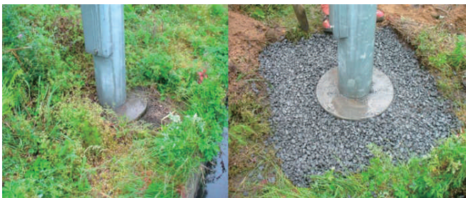
写真-5 照明柱基部環境改善（施工前・施工後） Photo.5 Improving Environment around the Base of the Pole
