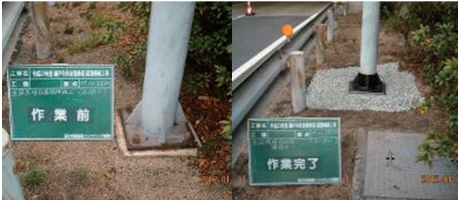
写真-4 液体ゴム防食補修（施工前・施工後） Photo.4 Repair of Corrosion Protection Coated by Liquid Rubber
