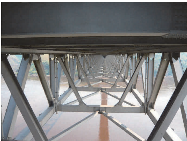
写真-4 補剛桁 Photo 4 Stiffening Girder
