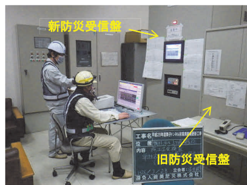
写真-7 防災受信盤の併設状況 Photo 7 The juxtaposition of existing/new disaster prevention reception board
