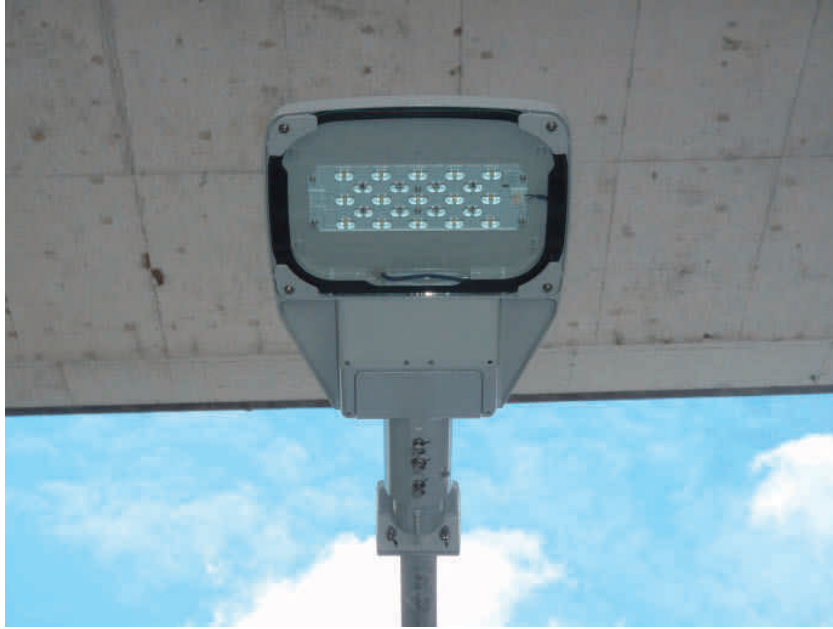
写真-8 LED 照明器具 LED lighting fixture
