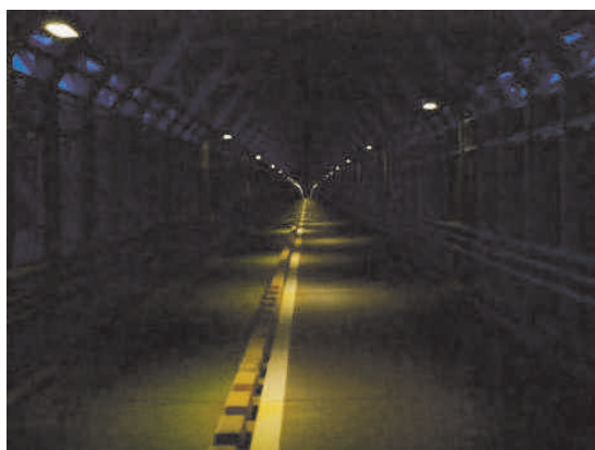
写真-3 蛍光灯照明器具（写真左）とLED照明器具（写真右）の夜間点灯状況 Photo.3 Fluorescence (left) and LED (right) lighting at night-time
