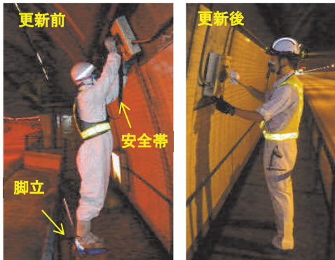
写真-3 火災検知器清掃状況 Photo 3 Cleaning of fire detector
