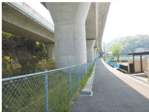
写真-2 市道に隣接した橋脚 Photo 2 Bridge piers adjacent to city road
