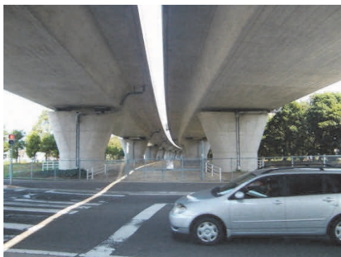
写真-1 橋脚と周辺道路 Photo 1 Rural road around bridge piers
