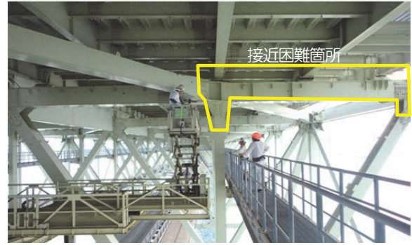
写真-16 明石海峡大橋鋼床版等の接近困難箇所 Photo 16 Hard-to-reach area underside of steel deck of the Akashi-Kaikyo Bridge
