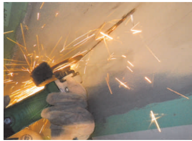
写真-5 溶接切削 Photo 5 Bead cut
