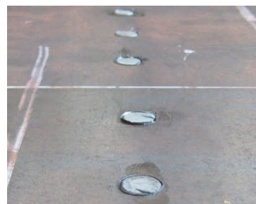
写真-1 TRS 施工後のデッキ上面 Photo 1 Upper side of the deck after repair
