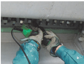
写真-7 TRS 締め込み Photo 7 TRS tightening
