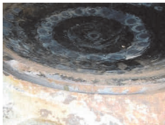
写真-4 下沓内部球面加工部の状況 Photo 4 Spherical surface inside of bottom bearing
