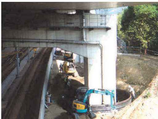
写真-6 HVa6P (東側) 掘削状況 Photo 6 Excavation around HVa6P (eastern side)
