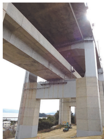
写真－11 HVa12P 柱部・梁部補強完了 Photo 11 After retrofitting at pier and beam, HVa12P
