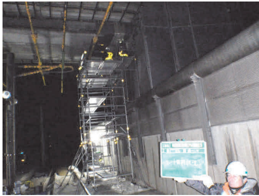
写真-4 JR 委託繊維巻立て作業 Photo 4 Fiber lining done by JR work
