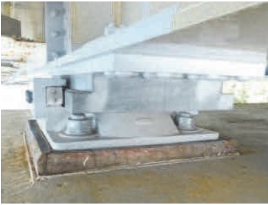
写真-7 支承補修後 Photo 7 Bearing after repair
