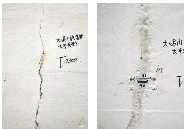
(a) N1A-1 (a) N1A-1 (b) N1A-2 (補修履歴有) (b) N1A-2 (with repair history)
