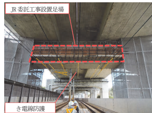
写真-3 JR 委託工事設置足場 Photo 3 Scaffolding done by JR work
