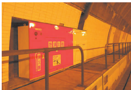
写真-7 更新後の舞子トンネル消火栓(SUS) Photo 7 Tunnel fire hydrant after renewal(SUS)
