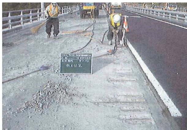
写真-2 断面補修状況 Photo 2 Section repair
