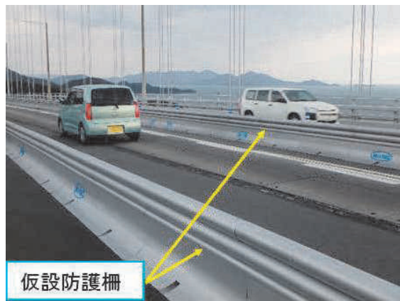
写真－6 仮設防護柵 Photo 6 Temporary protective fence
