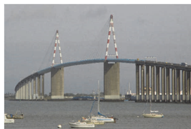
写真-2 Saint Nazaire Bridge
