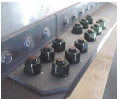
写真-13 T字形材連結 Photo 13 Connecting T-shape ribs
