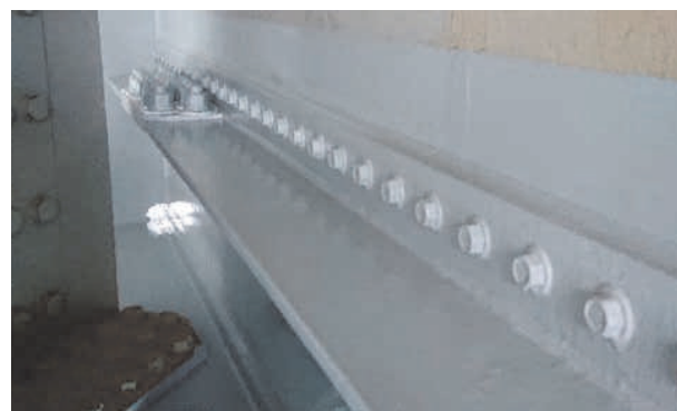
写真-14 施工完了 Photo 14 Construct completion
