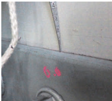
写真-16 肌隙計測 Photo 16 Gap measurement
