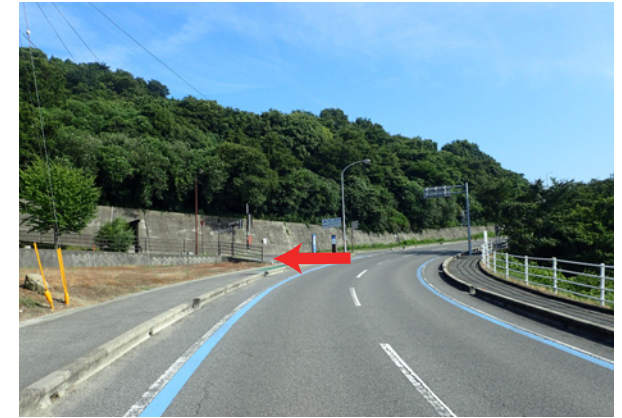
Ohshima Island side entrance and exit (motorized bicycle entrance and exit)
